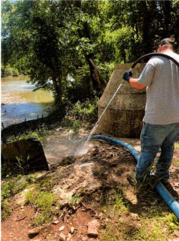
MH 1748 During Cleanup 5/1/2025
