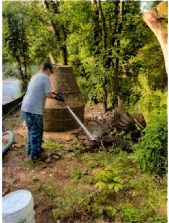
MH 1748 During Cleanup 5/9/2025
