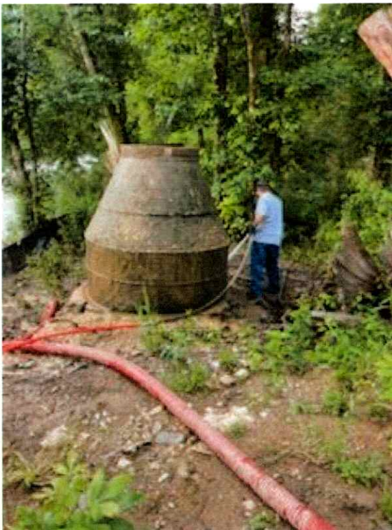
MH 1748 During cleanup – 5/29/2025
