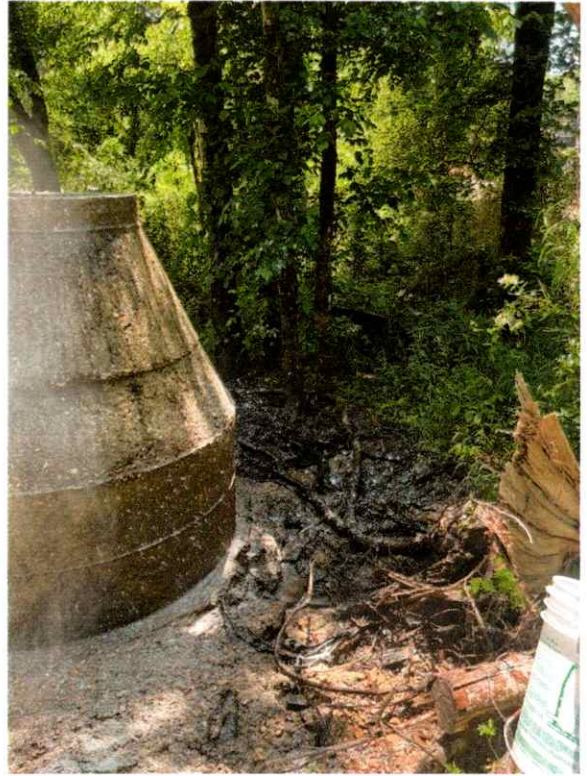
MH 1748 After Cleanup 5/1/2025
