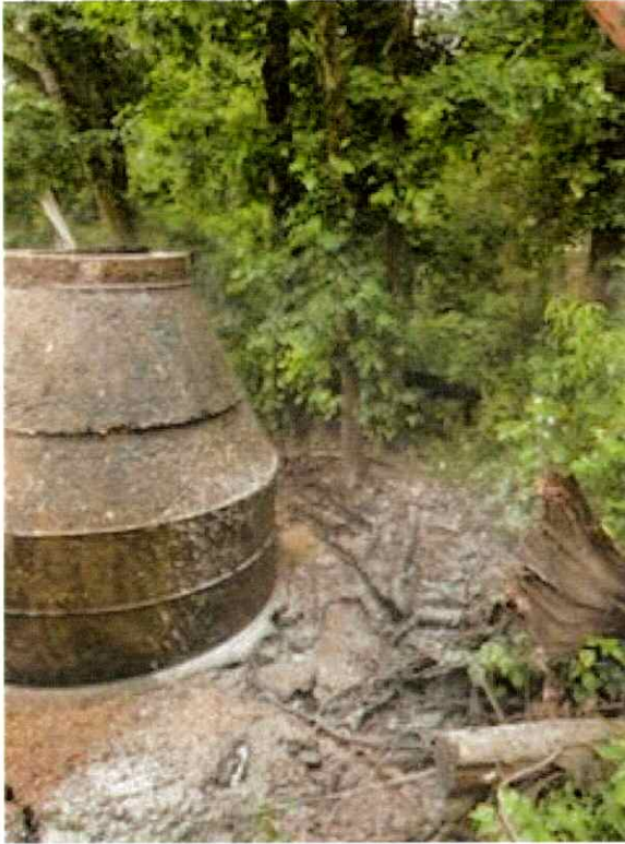
MH 1748 After Cleanup – 5/29/2025
