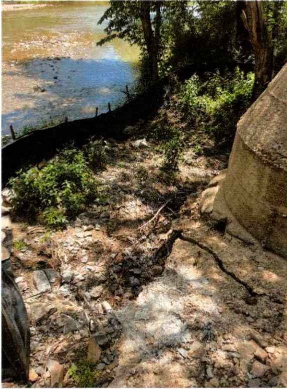
MH 1748 After Cleanup 5/1/2025
