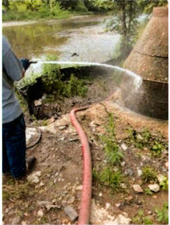
MH 1748 During cleanup – 5/29/2025
