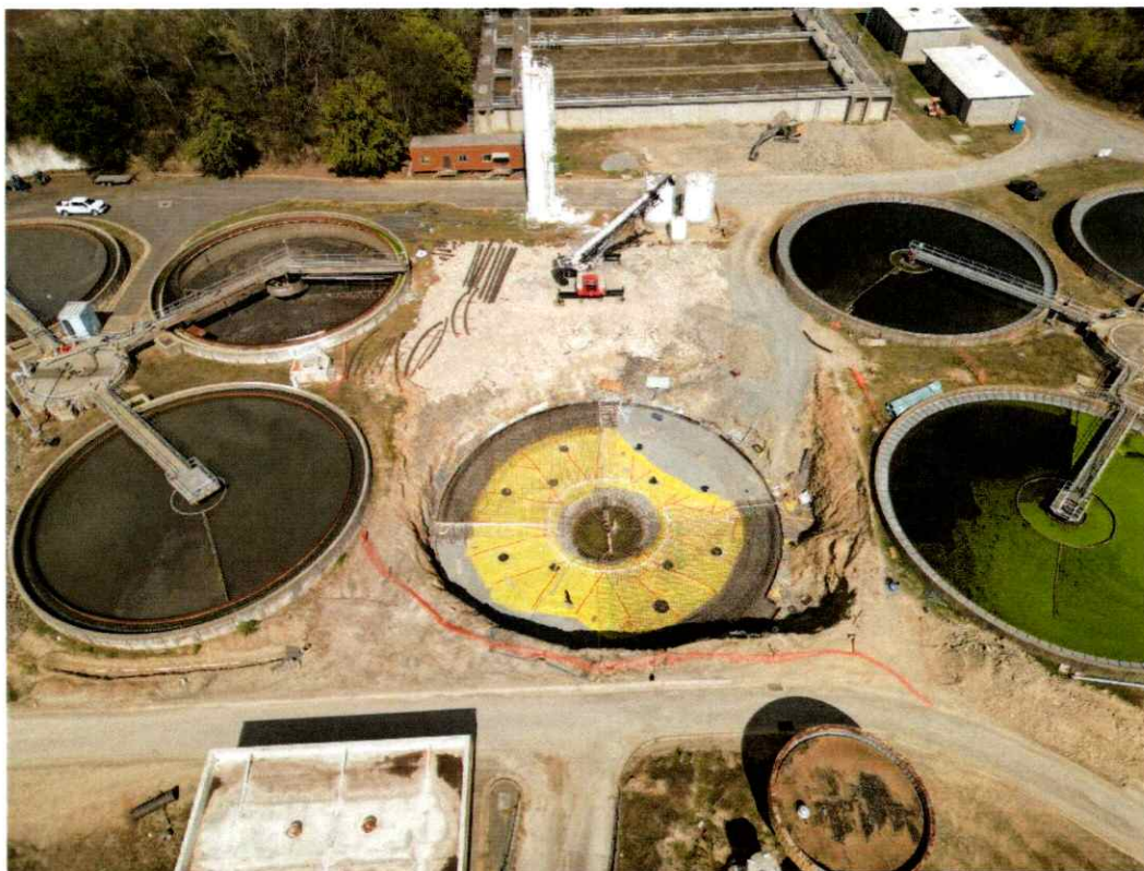
New 100 ft. Diameter Clarifier - Davidson WWTP
