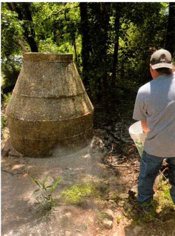
MH 1748 During Cleanup 5/1/2025
