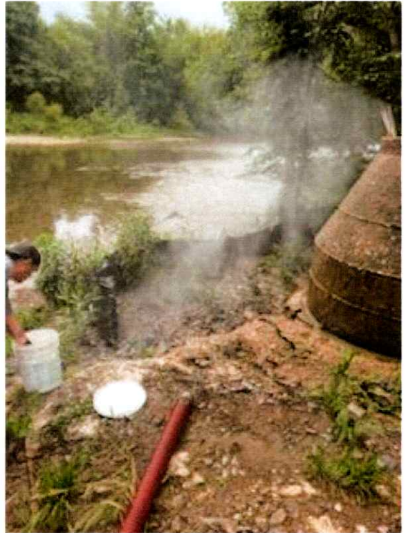
MH 1748 During Cleanup 5/9/2025
