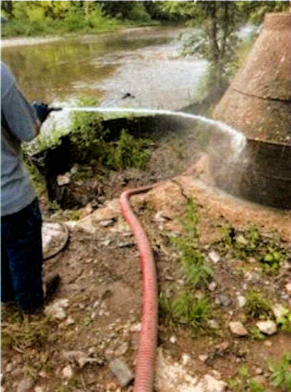
MH 1748 During Cleanup 5/9/2025
